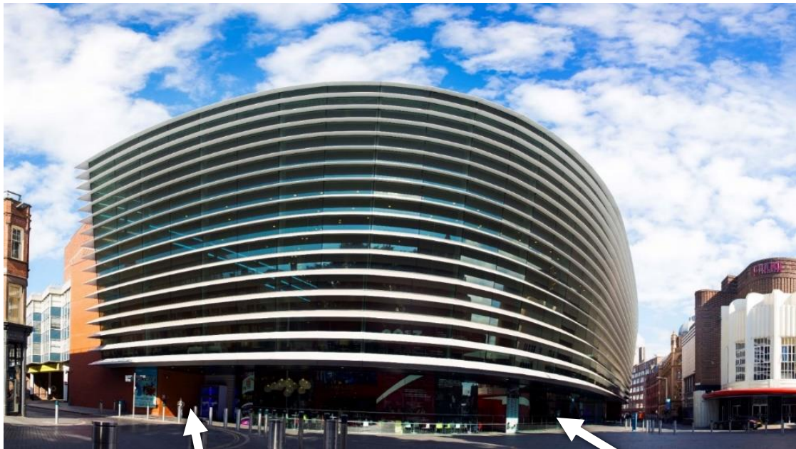
Halford Street Entrance
